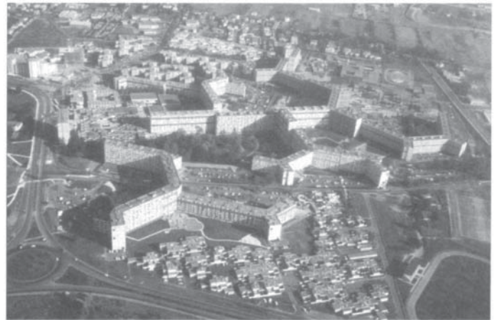
Fig. 10. Toulouse le Mirail , aerial view.
